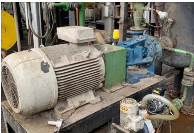
Bomba centrífuga Denver Orion 75/50.
